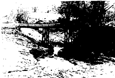
Dangerous county road bridge to be replaced by road structure four miles south; two east of Winside. Bridge replacement, $28,000.
